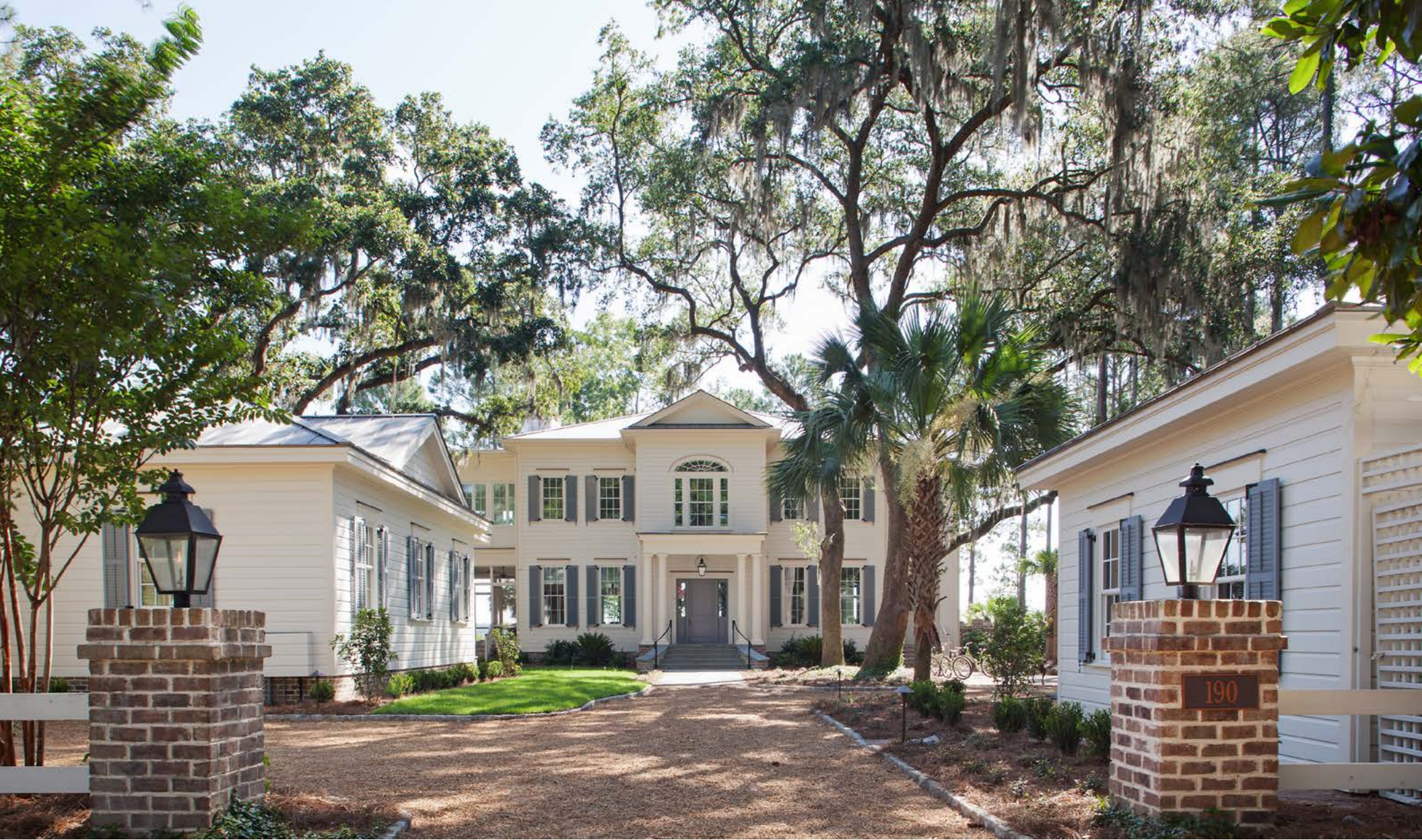
PRIVATE RESIDENCE Palmetto Bluff, South Carolina
